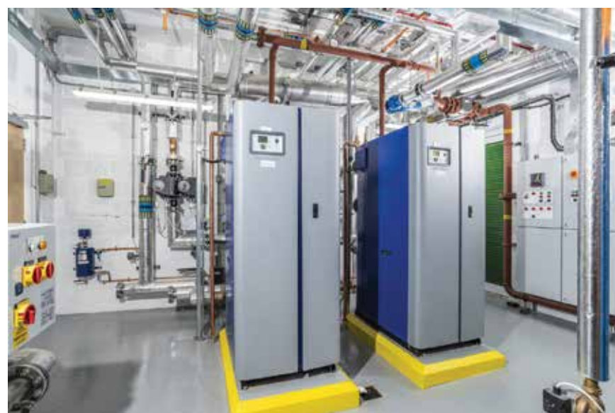
The use of a no flow boiler with twin return connections can combine low temperature (e. g. underfloor heating) and high temperature heating circuits.
