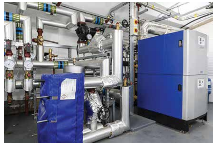
A plate heat exchanger delivers 'full' hydraulic separation and protects equipment from debris and pressure.
