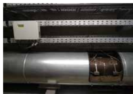
Fig. 3. Clamp-on metering at a major UK airport
