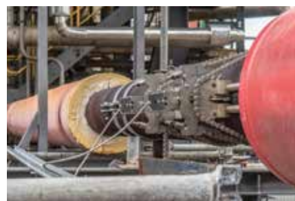
Fig. 4. Clamp-on steam measurement at major chemical manufacturing plant
