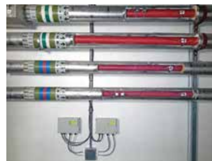
Fig. 2. Typical data centre installation showing clamp-on flow transducers and PT100 temperature sensors prior to re-insulating over the pipes.
